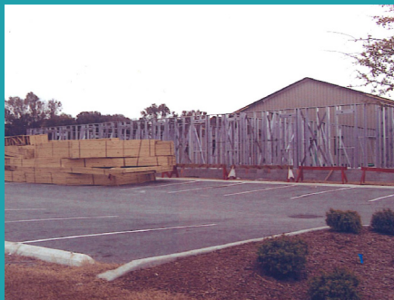
Night Shelter under construction - 2005
